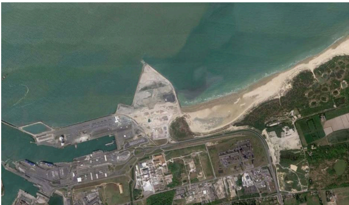
Construction of the port's expansion through land reclamation, between 2015 and 2017, Google Earth
